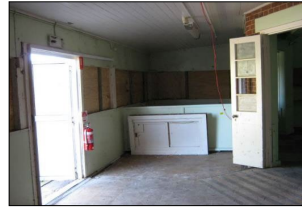
W Block: Floor tiles
