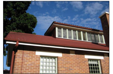
8737 C: External Skylight walls
