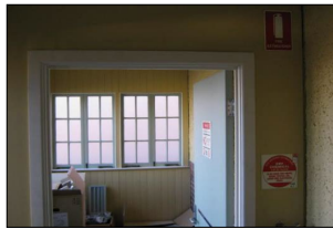
8757 A: K Block, foyer walls
