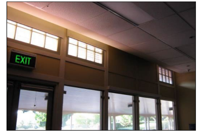
8739 B: C Block, upper wall panels
