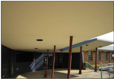
8730 A: B Block, Eave Soffits
