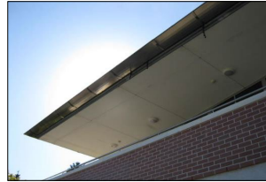
8748 A: H Block, veranda ceiling
