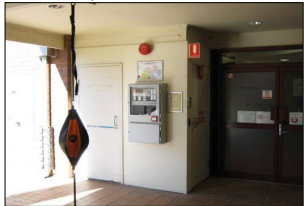
8741 A: G Block, entry walls
