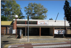
8741 C: G Block, vertical walls
