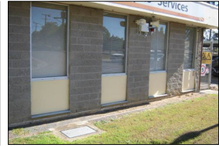
8766: V1 Block, window infill panels
