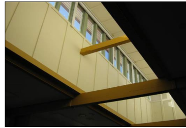
8737A: Internal Skylight walls
