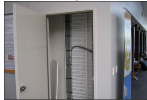
8749: H Block, Service room, walls
