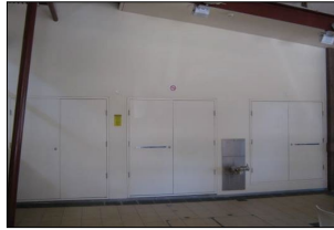
8759: L Block, external wall for Service room
