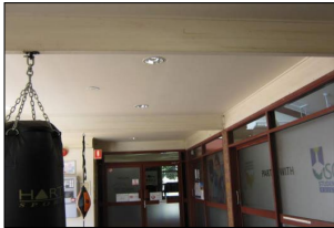
8742: G Block, entry ceiling
