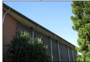
8748 B: H Block, eave soffits cladding
