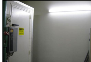
8747: H Block, Plant Room, walls
