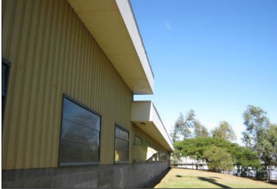
8765 C: V3 Block, eave soffits
