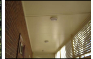
8751: P Block, veranda ceiling, 2 levels
