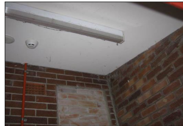
8735: C Block, C115, ceiling
