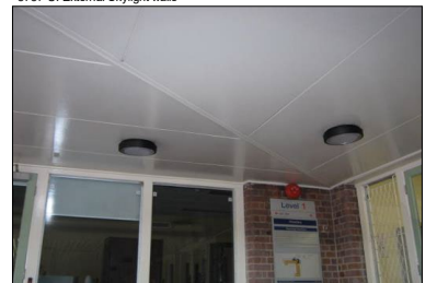
8738: C Block, veranda ceilings
