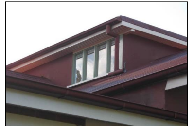
8737 B: External Skylight walls
