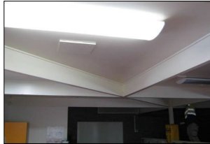
8746: G Block, internal ceiling, G112
