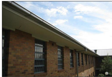
8730 B: B Block, Eave Soffits
