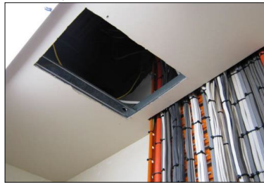
8731: B Block, Plant Room, ceiling
