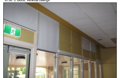
8739 A: C Block, C108, upper wall panels
