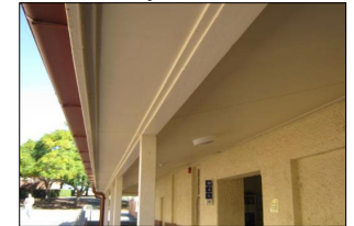
8752: M Block, veranda ceiling & eave soffits
