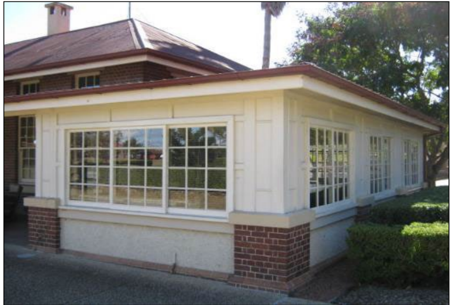
8771A: T Block, wall cladding, East end
