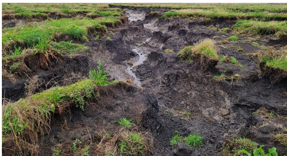
Figure 6 Example of flood damage in the Darling Downs from the January 2022 flooding. From the bottom of the washout to the top of the original soil is almost two metres deep.
